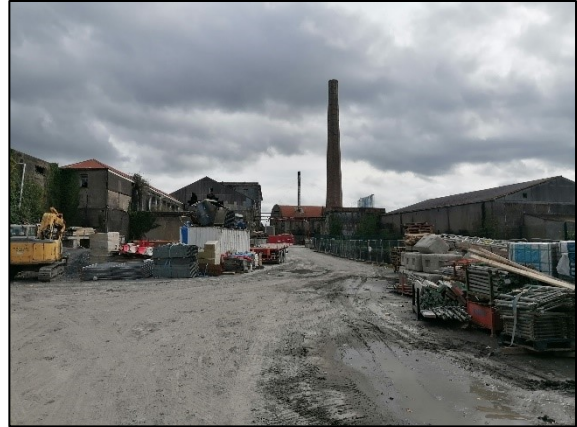
Plate 7.3-4 BL3 habitats seen from the Quarry site, used to store building materials
