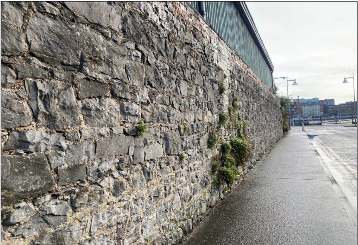
Plate 7.3-12: Stone Walls and Other Stone works (BL1) were recorded on the site in the form of existing boundary stone walls, pictured along NCR.
